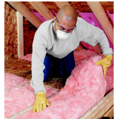
Batt insulation installation
