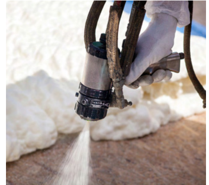
Spray foam insulation application
