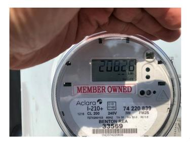
Above is the Benton REA Co-op Solar System Read on June 30, 2020, (last year's read) which you will need to retrieve from your last year's report. The Production/Member Owned meter read 20,826 kWh. This reading goes in Box #2 in the example form above.
